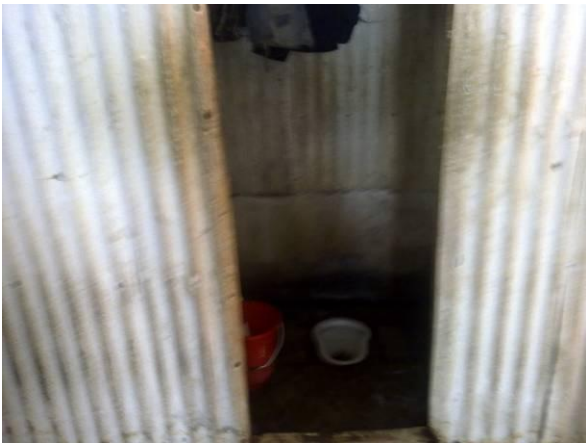
Toilets inside the barrack
