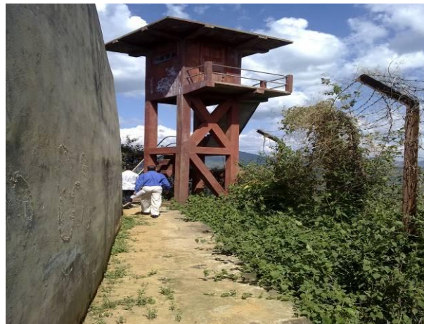
Security wall, watchtower and compound fence
