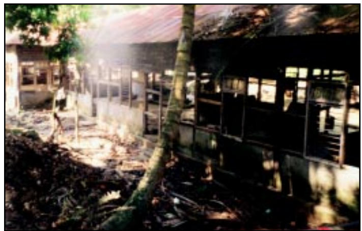
Destruction caused by Tsunami in Nancowry
