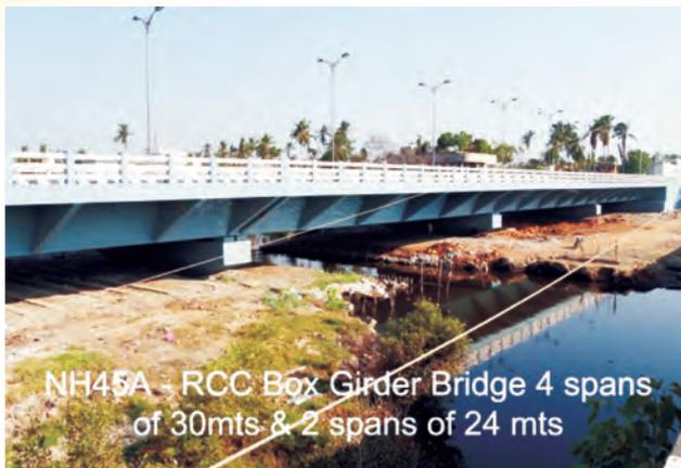
NH45A - RCC Box Girder Bridge 4 spans of 30mts & 2 spans of 24 mts
