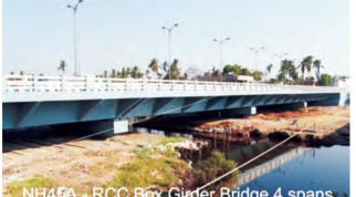
NH45A - RCC Box Girder Bridge 4 spans of 30mts & 2 spans of 24 mts
